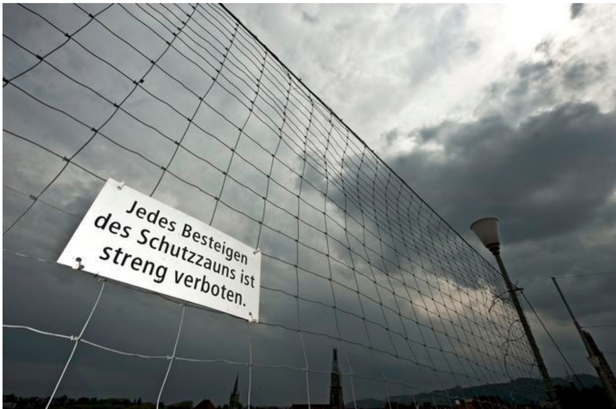
Figure 5: Fence at the Kornhausbrücke in Bern. The sign reads “every climbing at the safety fence is strictly prohibited” [source: Der Bund; 2011-04-28]
